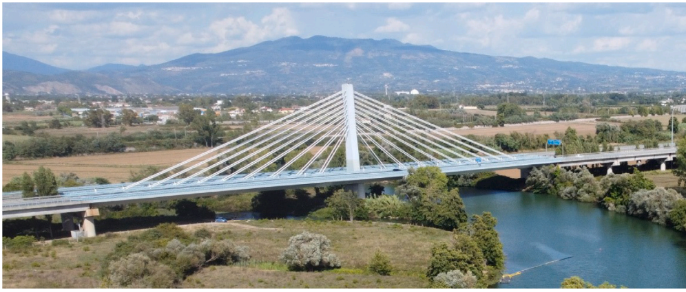
Fig. 11. Overview of stay-cabled bridge over the Garigliano river investigated in the present work.
