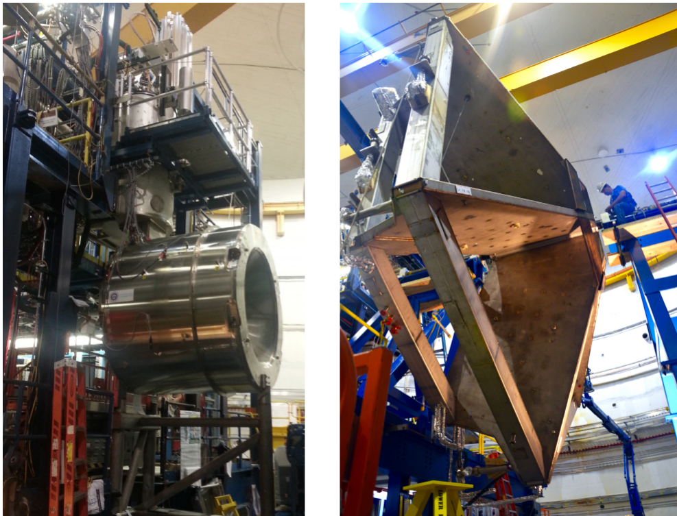
FIGURE 2.5: The CLAS12 magnet systems. Left: The fully assembled solenoid magnet including all cryogenic connections on the beamline at the beginning of cool down, before the detector installation. Right: The torus magnet with all six coils mechanically assembled in a common cryostat. The coil cryostat, which is fabricated from non-magnetic steel, has an outside width of 124 mm. The cross bars provide a cold (4.5 K) cryogenic connection of neighboring coils and counteract the out-of-plane forces to provide mechanical stability to the full magnet. Due to the large physical size of the assembled torus magnet, the final assembly of the magnet had to be completed in Hall B.
