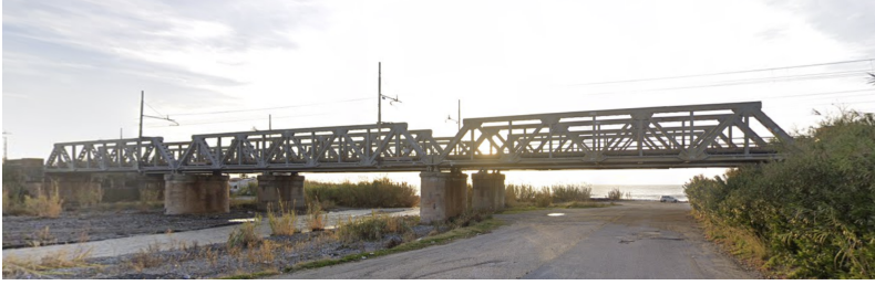
Figure 4.18: Overview of steel railway bridge investigated in the present study.
