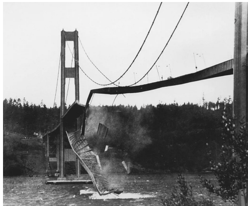
Figure 1.4: Collapse of Tacoma Narrows Bridge (1940) due to resonance phenomenon.
