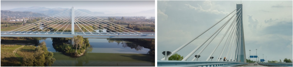
Figure 3.16: Overview of the cable-stayed bridge over the Garigliano river.
