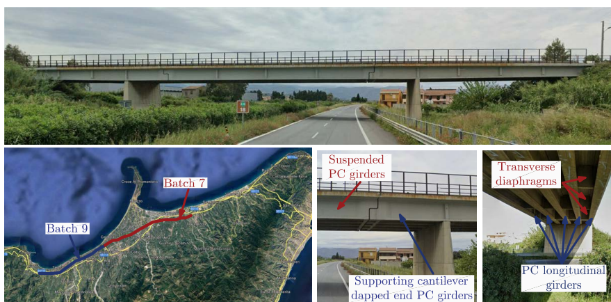
Figure 3.28: Overview of one of the A20 road overpasses representative of the series investigated in the present study.
