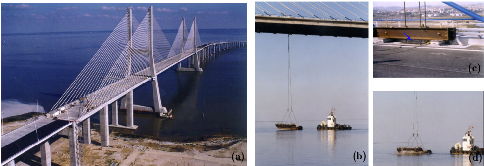
Figure 1.8: Free vibration test performed on Vasco da Gama cable-stayed bridge [38]: (a) overview of the bridge; (b) eccentrically suspended 60 ton barge; (c) starting cut of hanging Dywidag bar; (d) release of the barge.
