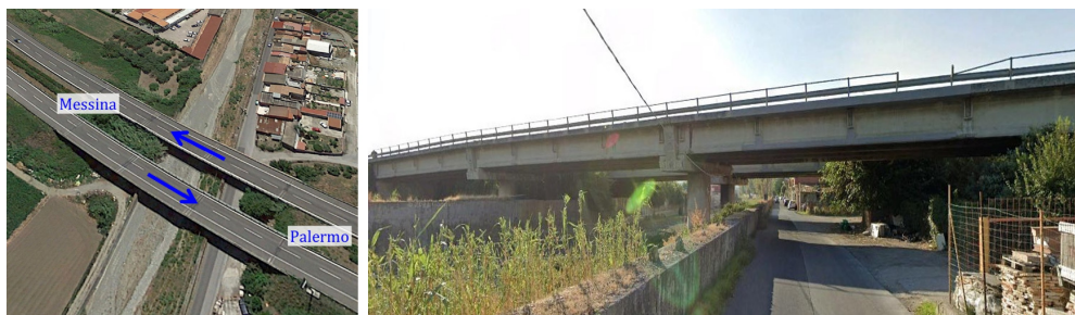
Figure 3.5: Overview of the Longano viaduct.
