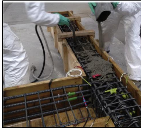
Figure 1.12. Electric arc furnace slag as aggregate for concrete production 93 .
