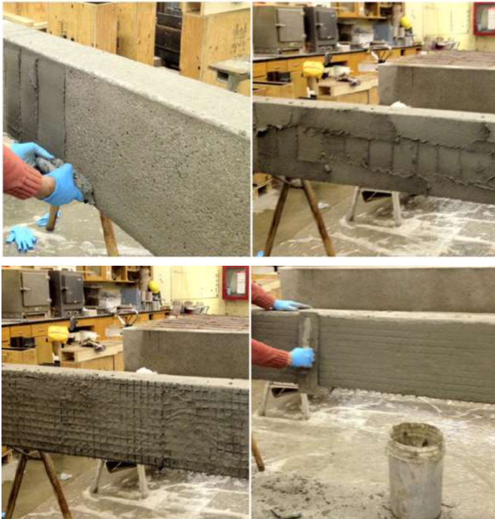
Figure 4.2 Example of FRCM application
