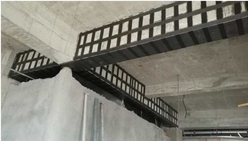
Figure 4.1 Example of FRP strengthening applied on a concrete substrate
