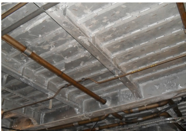
Fig. 2. Deck panel made of AA 5083.
