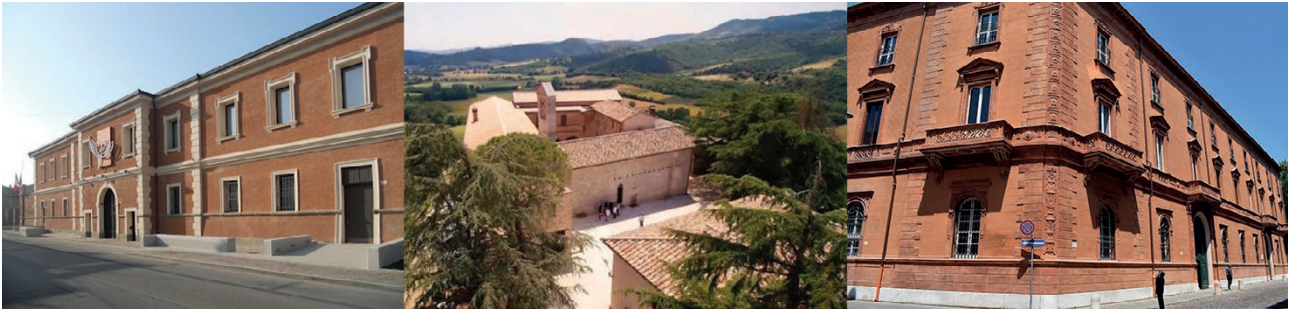
Fig. 1 | Buildings with GBC Historic Building certification: 1) National Museum of Italian Judaism and the Shoah, in Ferrara, 2) the stables of the Benedictine monastery of the Rocca di Sant'Apollinare (PG), 3) palazzo Gulinelli in Ferrara.
