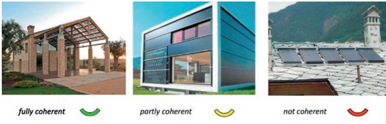
Fig. 5 | Different levels of “System materiality” coherency (photo: M. C. Munari Probst, C. Roecker).
