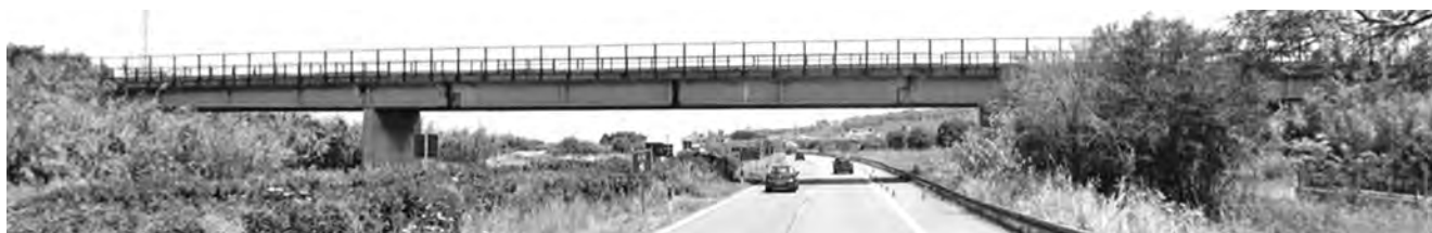
FIGURE 11 View of the overpass
