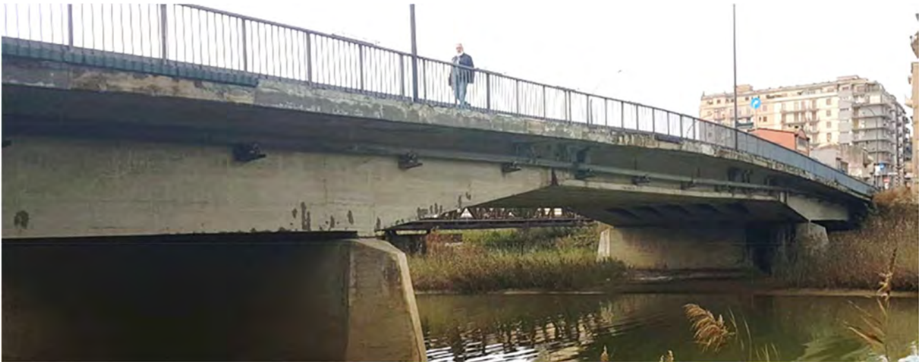
FIGURE 4 View of the bridge
