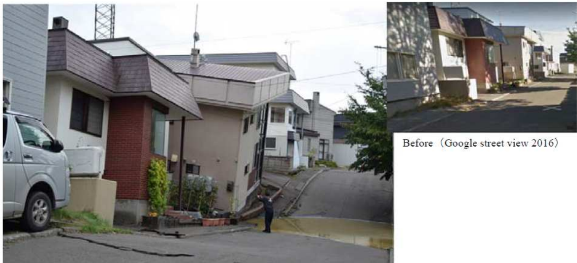
Figure 1 – Deformations induced by the phenomenon of liquefaction following the Hokkaido Iburi-East earthquake (2018) (Sapporo City Office 2018).
