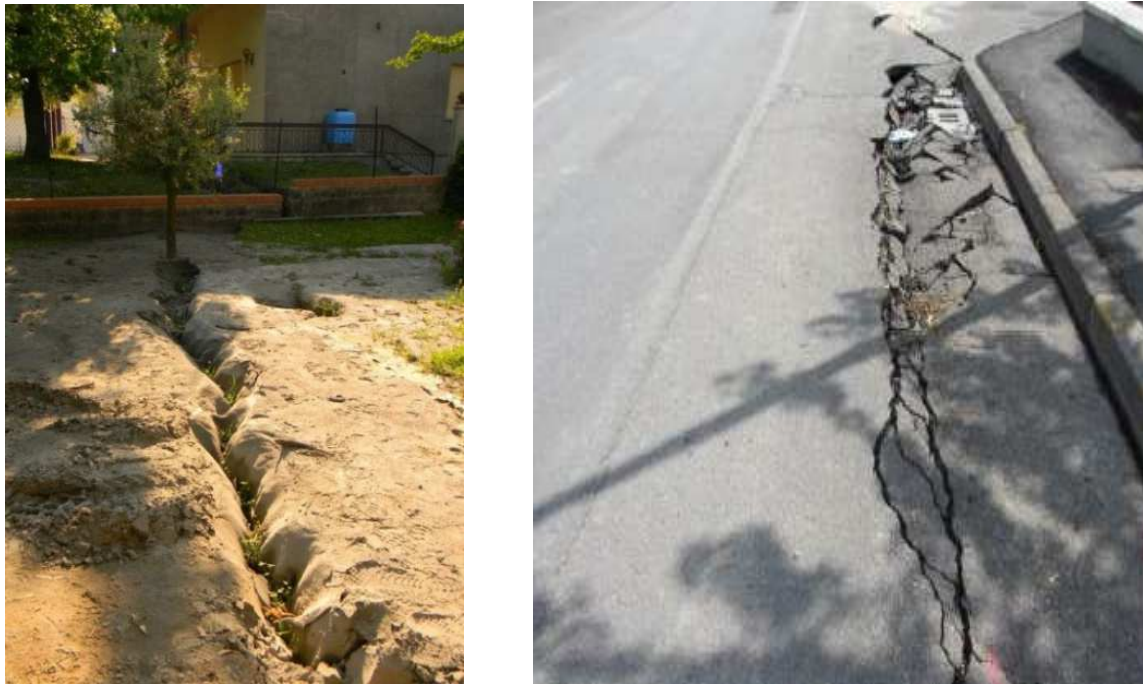
Figure 3 – Effects of the liquefaction phenomenon following the 2012 Emilia Romagna earthquake (Tonni et al. 2015).
